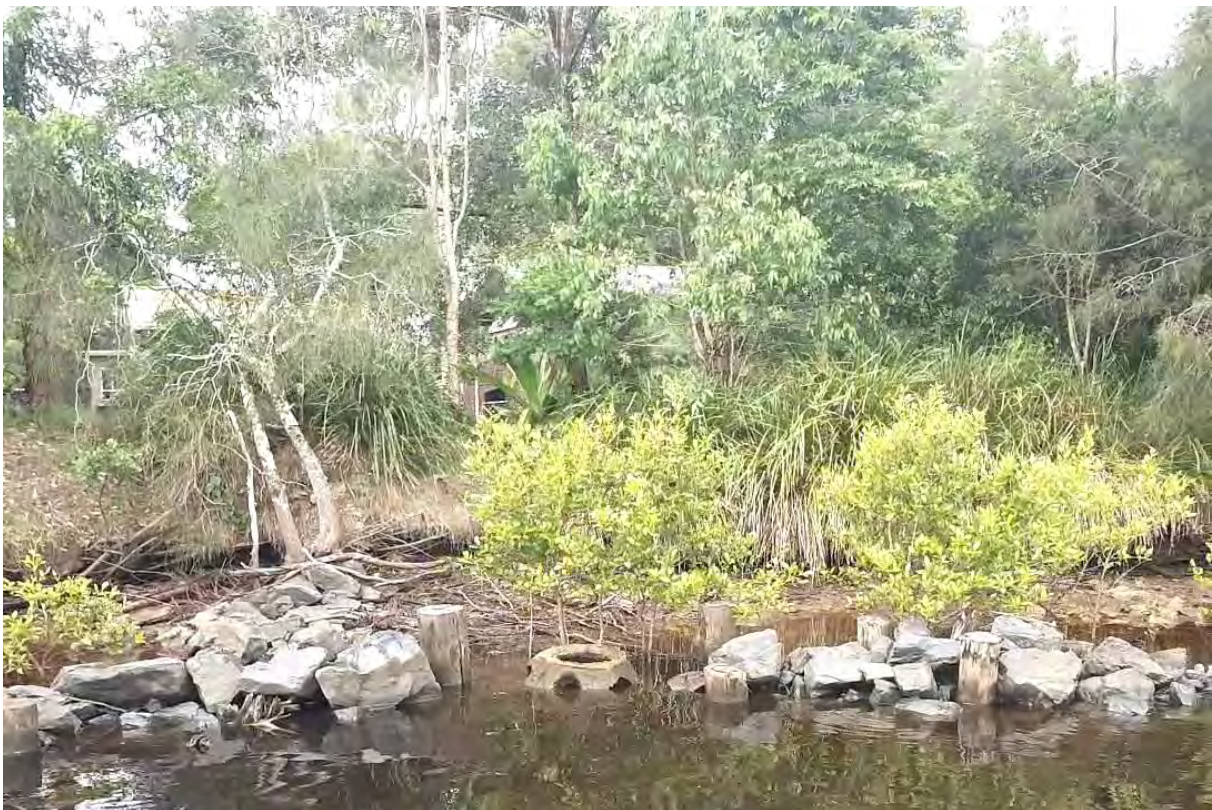
Figure A-25 Mangrove re-establishment behind rock fillets, Newry Island
