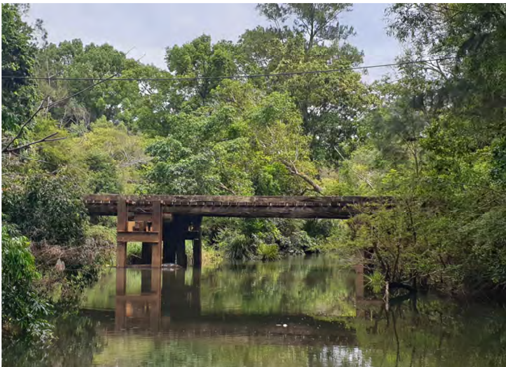
Figure A-4 Bowraville Road Bridge, near Tidal Limit of Kalang River at Brierfield (captured High Tide, 7 December 2021)
