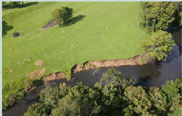
Aerial and drone photography allowed the project team to inspect the extent of issues such as riverbank erosion.
