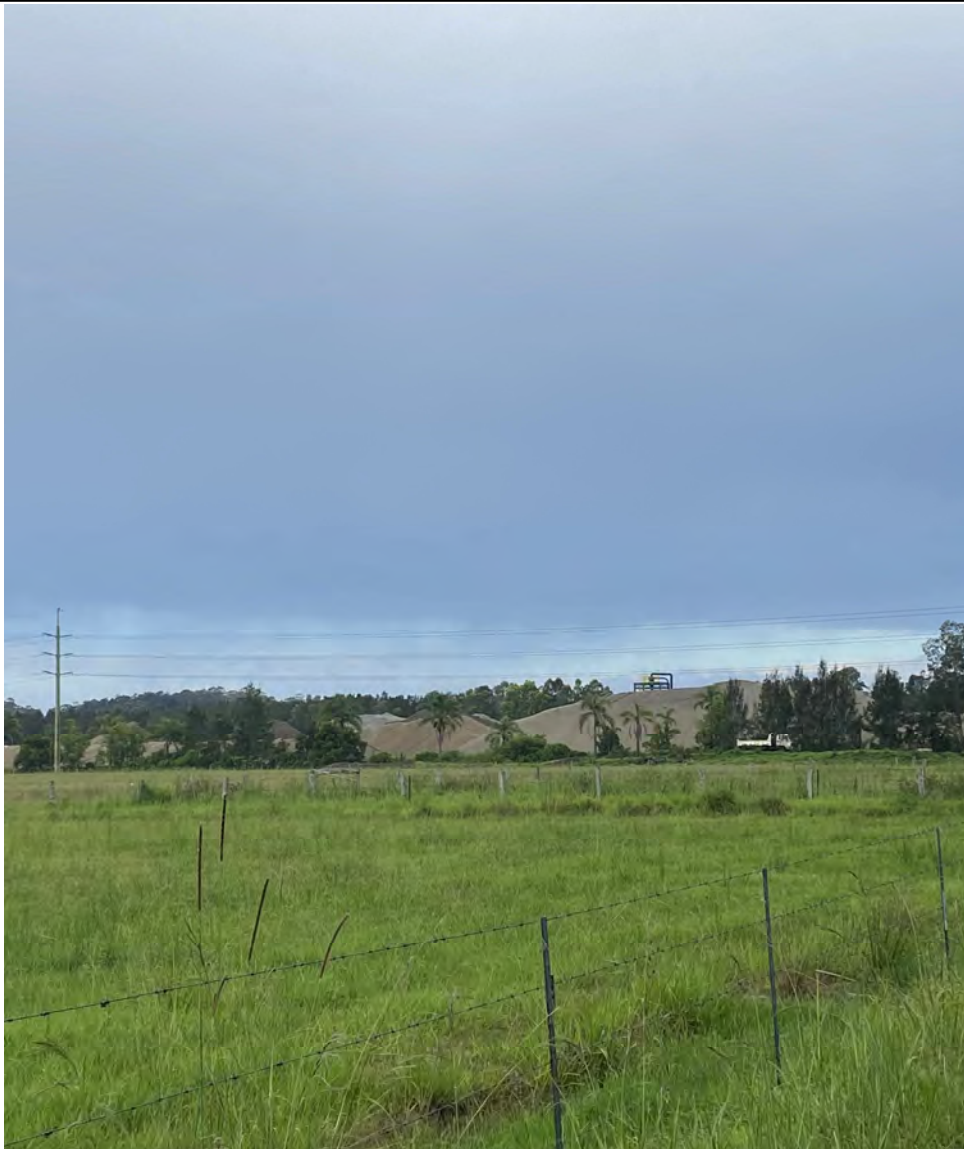
Figure A-5 Facility at Repton used to Process Sand Extracted from the Bellinger River downstream of the Pacific Highway
