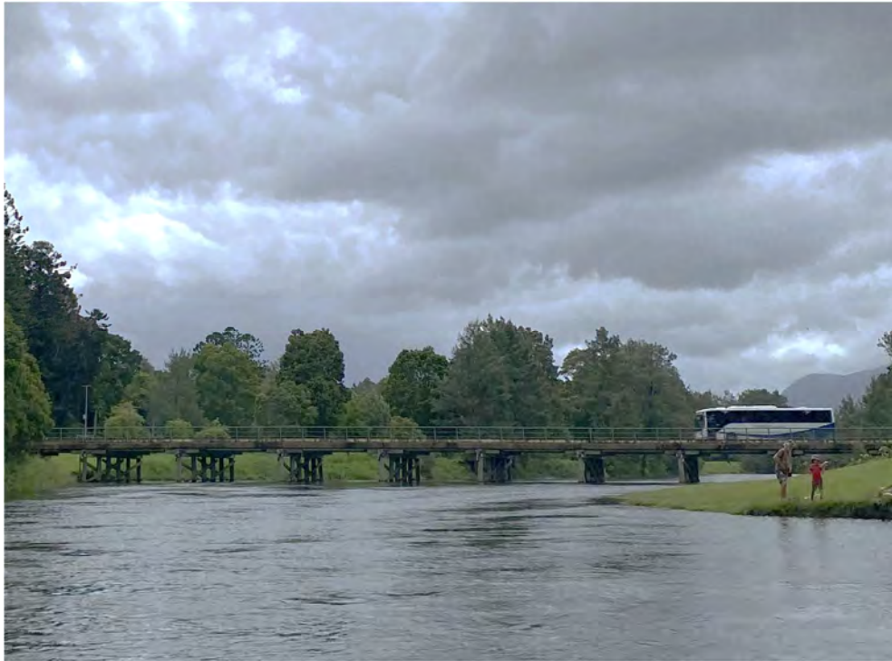
Figure A-3 Lavender Bridge at Bellingen, near Tidal Limit of Bellinger River (captured High Tide, 6 December 2021)
