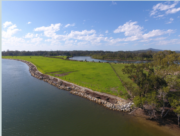
Image: Rock revetment at Newry Island
