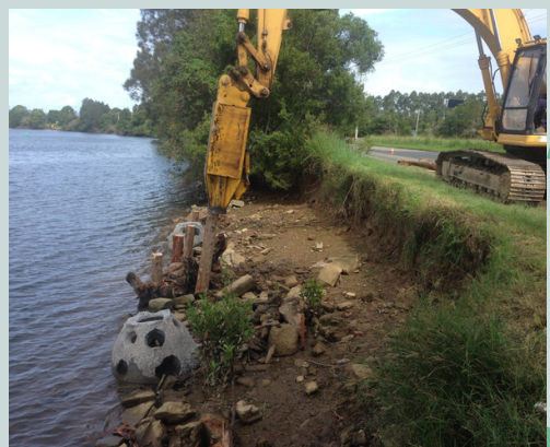
Image: Driving pins for rock fillet works at Mylestom
